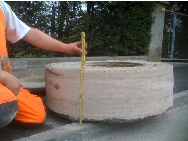
Bohren Belag 5 cm, Rest Beton
